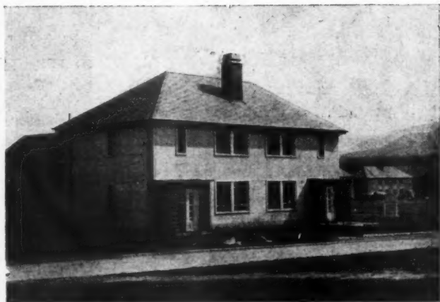
1947. AN ORLIT PREFABRICATED CONCRETE HOUSE WITH WALLS COLOURED EXTERNALLY WITH CEMENTONE No. 1 PERMANENT COLOURS.
