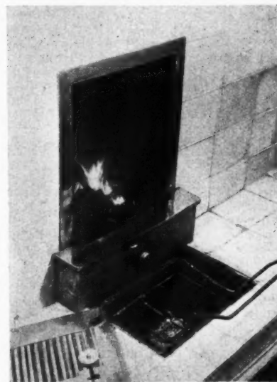
Closeable open fire developed by the Coal Utilization Research Association. The air to be warmed and fed to the upper floors is fed to the fire through the hearth or from outside the house, and the hopper holds a full week's production of ash.
