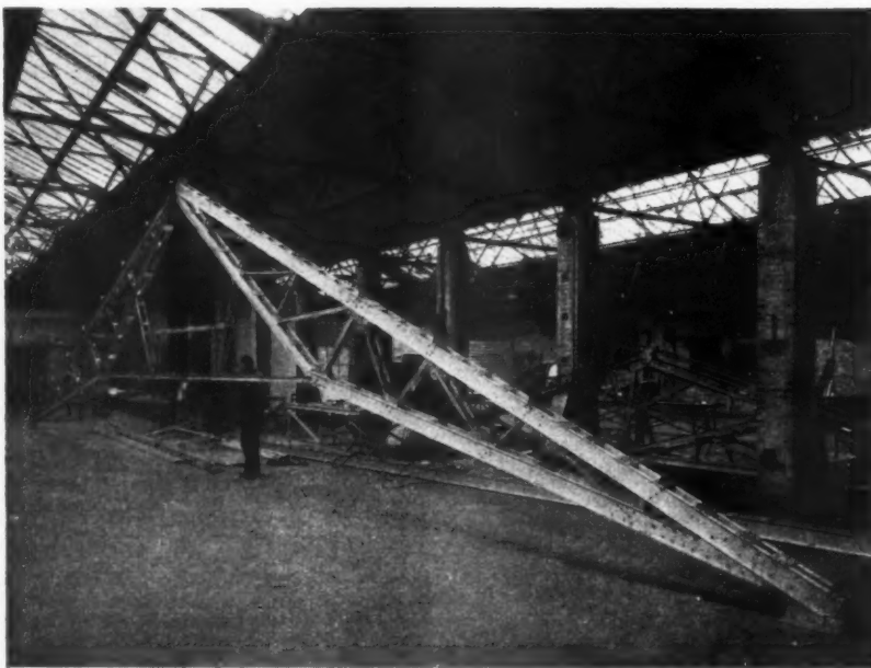
Fig. 1. 60-ft. span light alloy truss for a cinema at Rye. This particular example weighs about 8 cwt. (Structural and Mechanical Developments, Slough. Stand E 96.)
