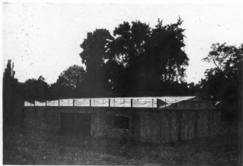
Fig. 9. S.M.D. transportable building in aluminium alloy. Clear floor space 72 ft. by 35 ft.
