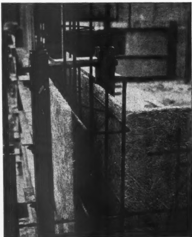
"Gypklith" as permanent shuttering. Junction of transverse wall with external wall showing reinforcement in position, ready for pouring concrete. Reproduced by permission of the "Cement and Concrete Association"
