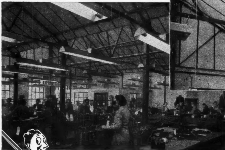
Knitwear Factory for R. J. & A. R. Pitchers Ltd. (An associate of the Jaeger Co. Ltd.) Godalming, Surrey. Roof and gable walls lined by Specialised Construction, during occupation by the Hadley Clip method.
