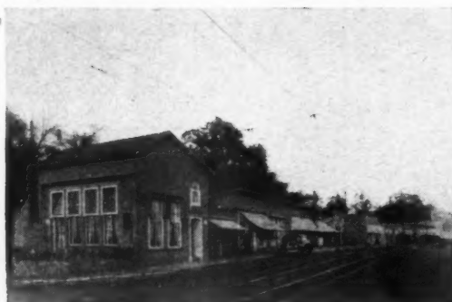
Three types of temporary one-storey shops, built in the devastated centre of Nijmegen to maintain the town's position as a regional shopping centre. The upper type is of white-washed concrete blocks; the two lower types of yellow and red brick respectively.
