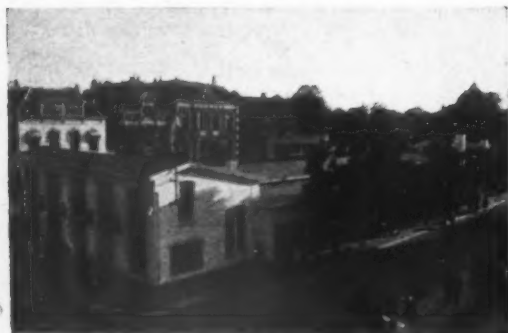
Three types of temporary one-storey shops, built in the devastated centre of Nijmegen to maintain the town's position as a regional shopping centre. The upper type is of white-washed concrete blocks; the two lower types of yellow and red brick respectively.
