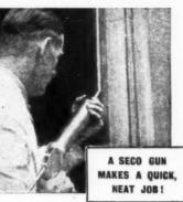
The Seco hand caulking gun can be worked with ease, speed and precision ; it reduces wastage and labour costs to a minimum ; it forces the Secomastic into the joint, ensuring uniform and deep penetration.
