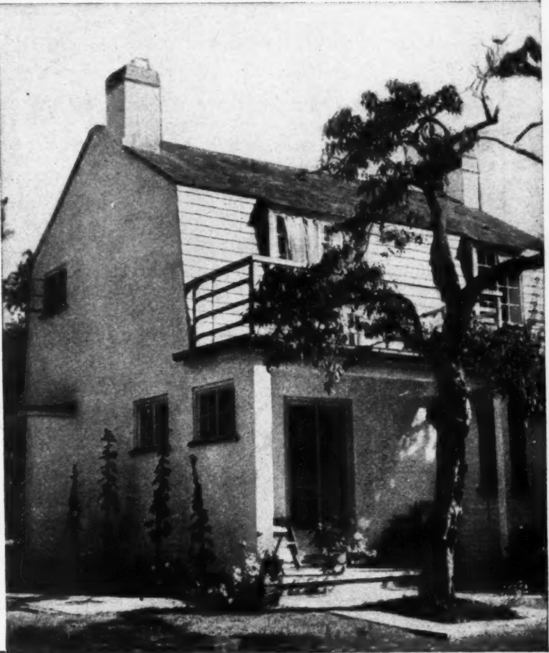
House at Crown Lane, East Burham, Bucks, roofed with Colt Shingles.
