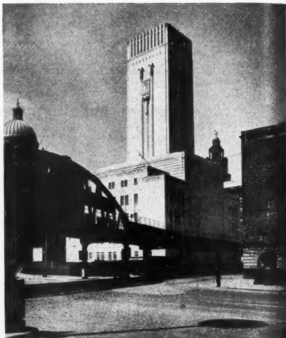
Mersey Tunnel, George's Dock Ventilation Building. A new problem in architectural design was offered in the several buildings, of which this is one, constructed for the purpose the name implies; that is, to house the machinery and plant and make provision for efficient ventilation of the recently constructed engineering feat beneath the river—Queensway, the Mersey Tunnel. All these buildings have been designed by Mr. H. J. Rowse, and in their semi-skyscraper form contribute a new feature to the Merseyside skyline. Note the complete lack of fenestration in the shaft. This particular building is constructed with a concrete encased steel frame, reinforced concrete ducting and Portland stone external facing.
