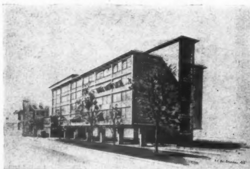
A project for the Treatment Block of a Children's Hospital, designed by Herbert Thearle. The site is an old burial ground, so the building has been designed to cover as little of the ground as possible to avoid the cost of re-interring the bodies.
