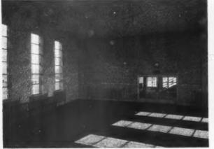
The assembly hall at Ecclesfield School, by Sir John Burnet, Tait and Lorne. The rear wall is lined with acousti-celotex in 24-in. by 12-in. panels in natural colour. Walls and ceilings are white, and dados and radiators pale blue. The floor is oak block.
