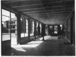
Entrance hall of St. Audrey's School, Hatfield, by H. V. Lobb. Fair-faced brickwork is used, and a solid floor with a wood-wool ceiling to minimise acoustic resonance. The entrance is treated as the enlargement of a corridor.
