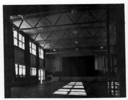
The assembly hall at Bourne School, Middlesex, by Howard Lobb. The ceiling is of wood wool with the bays nearest the stage plastered to produce an acoustic reflection. At the entrance end the wood wool is distempered only, in order to leave its sound absorbent qualities unimpaired. The curtains on the windows are also sound absorbent, and the welded roof trusses serve to break up sound waves.
