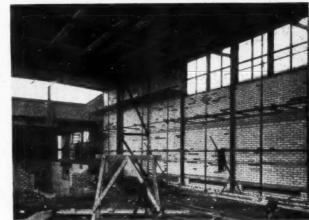
Right, two stages in the construction of a steel framed school with brick panelled walls. The centre photograph is of the assembly hall at School, Bourne Middlesex, the lower shows the dining block at Field End Road School, Middlesex. Both were designed by H. V. Lobb.
