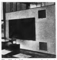
The Weatherfoil apparatus referred to in the article. After installation the air intake and discharge grills alone are visible.
