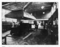
The kitchen at Bourne School, Middlesex. The equipment consists of gas-fired steaming ovens and boiling pans, centrally grouped to minimise labour. There is a hot cupboard on the kitchen side of the serving hatch.
