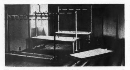
Three types of school coat rack. The one in the foreground is on castors and mobile. On the right is a nursery school day bed, and in the rear a rocker. All are of steel tubular construction.
