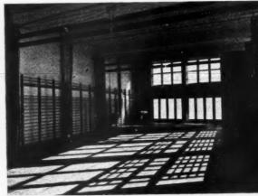
Gymnasium at Scalby School, by F. X. Velarde. The floor is of wood strip running across the short side of the room, and is best maintained with a non-slip preparation. It is desirable that the gymnasium floor should not be used for other activities.
