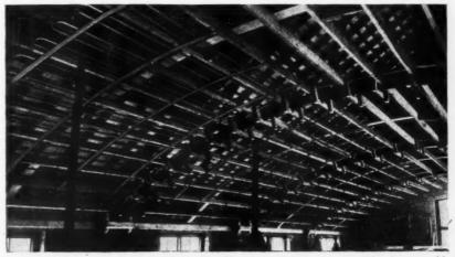
A heating layout for a school assembly hall. The photograph shows a panel heating assembly in a suspended ceiling and the methods of fixing the coils.
