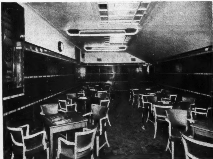
Low temperature electric panel heating used behind timber panelling. As can be seen in the photograph, the complete wall board veneer panelled heaters are flush with, and indistinguishable from, the remainder of the panelling in the room.
