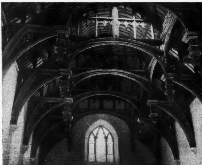
The restoration of Lambeth Palace after its war damage is described in a news note on page 549. The photographs show the work that has been done to Juxon's Great Hall which was badly burned. Right, the restored hammer-beam roof; above, an exterior view. The old grey slates have been replaced with tiles.
