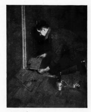
THE capacity of certain of the synthetic resins to soften under the influence of heat is turned to good account in the laying of SEMASTIC DECORATIVE TILES. Nothing in this world is completely square or perfectly straight apart from theoretical conceptions, and whilst the "tolerances" of engineers are measured in thousandths of an inch, much larger fractions must in practice be tolerated by the architect.
