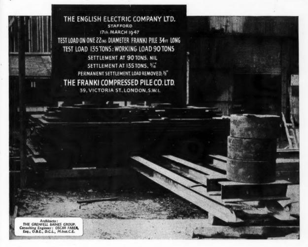
Actual photograph of a load test carried out on one Franki Pile, picked at random from the 405 installed on this particular site. The fact that such a concentrated load can safely be carried on a single Franki Pile is ample proof that
