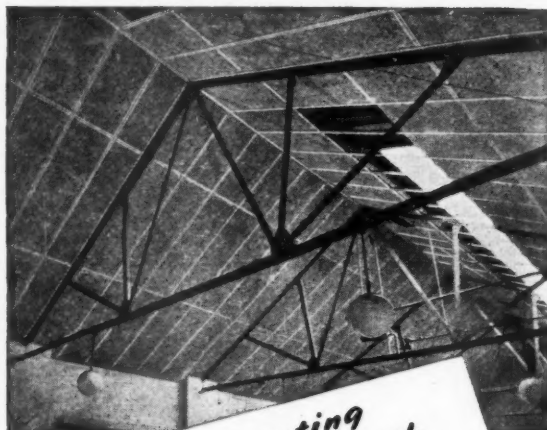
1" wood wool slabs carried on light gauge steel tees.
