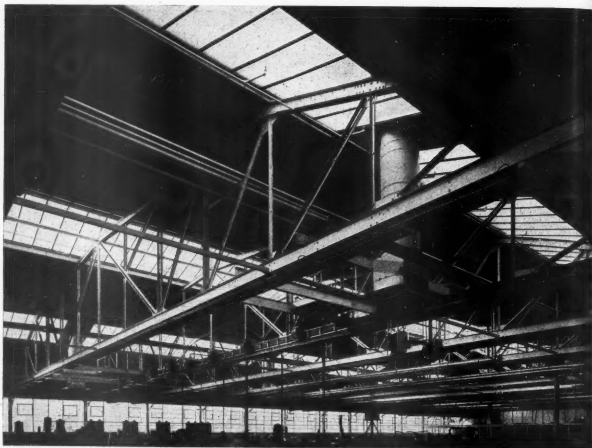
Above, the interior of the production shop, showing the 127 ft. roof truss. Below, the west elevation of the shop with projecting lavatory blocks and staircases.
