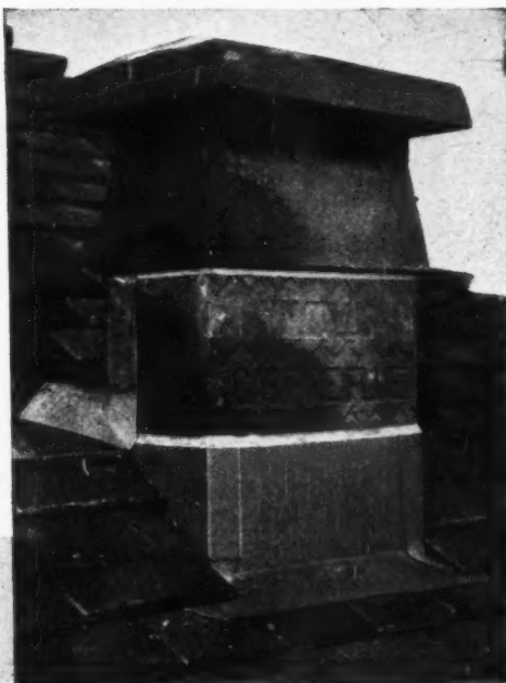
Two recent and widely differing examples of chimney flashings in sheet lead.
