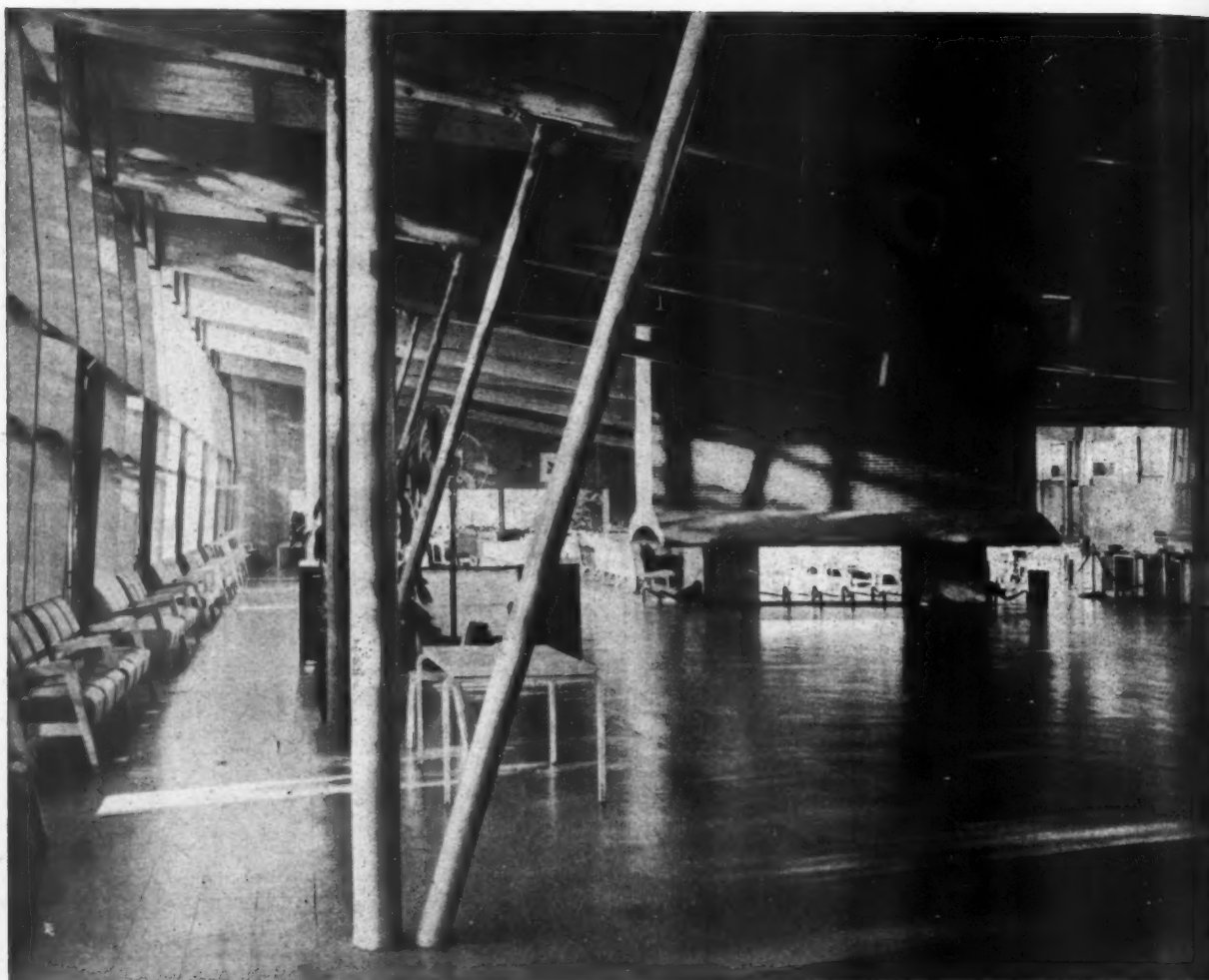
The lounge. The steel columns, supporting the laminated beams, contain the electrical connections for the fans, water cooler and lights.
