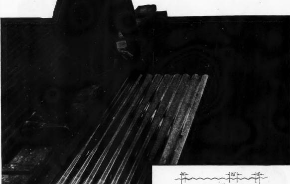
Corrugated "Perspex" acrylic sheet can be fixed as easily as normal corrugated sheet, using ordinary hook bolts and washers. Made in 9 different profiles, and available in lengths from 3 feet to 7 feet in intervals of 6 inches.
