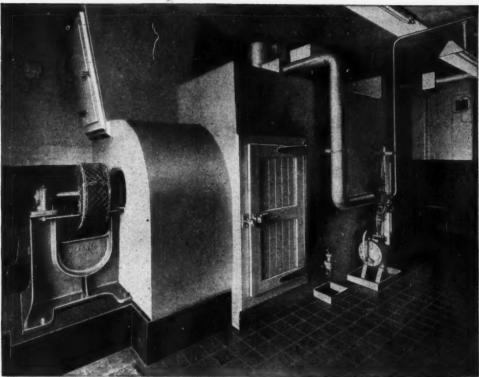
Where air-conditioning plant has to be installed, adequate and convenient space should be provided for refrigerating machines and bulky equipment such as that shown. The siting of all this is important, while the construction and layout of the air ducting can only be satisfactory and economical if it is planned by the Architect and Refrigerating Engineer working in collaboration.
