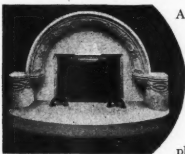
Cast stone made with Snowcrete is invaluable for interior decorative effects as well as for exterior reliefs such as windows and doorways.
