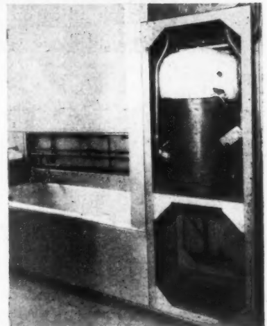
Above, the kitchen unit, which is backed by the bathroom unit, right and bottom. The photograph, right, shows the plumbing duct and the hot water tank, with the cold water tank immediately above.
