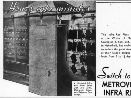
This Infra Red Plant, installed at the Works of Messrs, T. Crompton & Sons Ltd., Ashtonin-Makerfield, has enabled them to reduce the paint stoving time of their week's output of door locks from 5 to 14 days.
