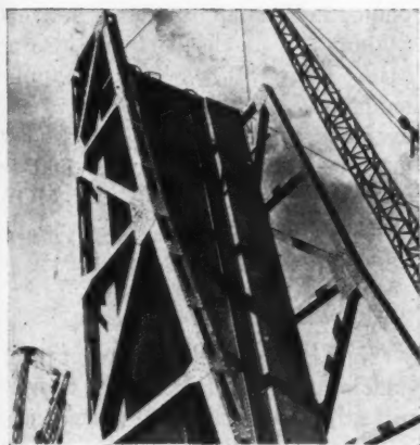
A drawing was published in the JOURNAL for July 1 of the projected aluminium bridge at Alvida, Quebec, which was expected to be the first all-aluminium bridge to be completed in the world. The Canadians have now found themselves forestalled by the opening last week, by the Minister of Transport, of the new aluminium alloy bascule bridge at Sunderland. The photograph above shows part of the bridge under construction. Built as part of the Port of Sunderland Improvement Programme it spans the junction between the Hudson and Hendon Docks. Mr. W. H. S. Tripp, Engineer to the River Wear Commissioners, was responsible for the detailed design and execution of the work, and the superstructure was designed by Mr. F. J. Walker, Chief Civil Engineer of Head, Wrightson & Co. Ltd., who built the bridge.
