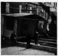
Fitzmaurice: "At the end of the line a house comes out every twelve minutes." The British aluminium factory-made house: one section as it comes off the assembly line being manœuvred on to its brick foundations.
