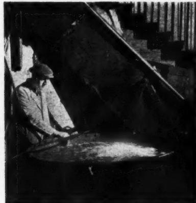
These photographs show work in progress in the now-abandoned shot-tower on the South Bank of the Thames. Left, pouring the molten lead through a sieve at the top of the tower. Right, the tank at the bottom which receives the falling shot.
