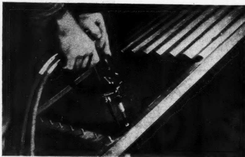
The Nelson gun welding studs for fixing corrugated sheet.
