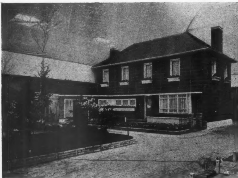
The Unity house completed save for interior decoration, in 50 hours by 20 tradesmen. The walls are precast concrete slabs erected "dry", clipped and wired to both faces of the reinforced concrete framing with a 6" cavity in between them. The edges of the outer slabs have a ship-lap joint made watertight by pointing with a mastic gun.
