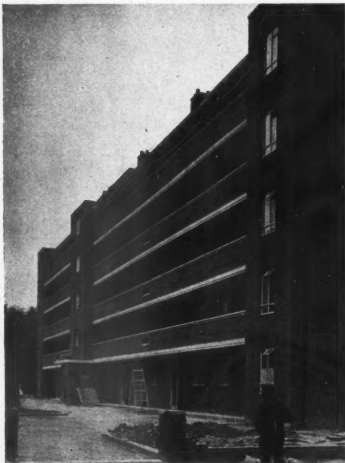
WOODBERRY DOWN ESTATE, STOKE NEWINGTON Left, one of the five-storey blocks of traditional brick construction with concrete floors. Top, the first eight-storey blocks (more fully illustrated in the JOURNAL for March 3). It is of monolithic concrete construction, with access by lifts and stairs. Above, the site plan. Altogether 1,765 families are accommodated on a site of 64 acres.
