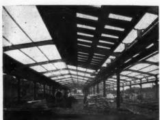
Multi-Span Ridged Arched Welded Construction
