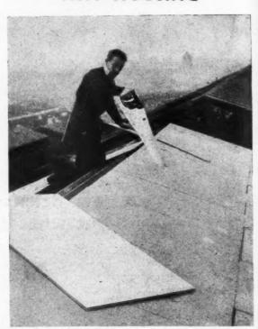
THE photograph illustrates the use of WEYROC as roofing on a housing estate. Sheets of WEYROC were used as sarking and copper-sheeted. A striking example of the way in which WEYROC is speeding the building trade!
