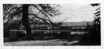
GENERAL.—A prefabricated unit system of school construction. This prototype three-classroom unit was built at Hatfield for the Herts County Council. It is con-sidered that similar units, on a flat site, could be put up in about six weeks.
