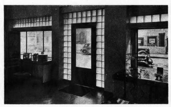
URING the day, natural light is diffused over the ground floor, and well into the basement through the stallboards. At night, from outside, the premises glow with light. Space heating is conserved in winter, summer heat and glare excluded, and traffic noise minimised.
