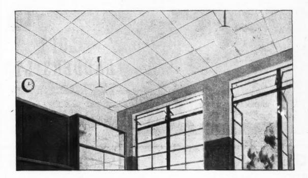
A new development in the fixing of insulation boards makes it possible for them to be fixed securely to teesections without exposing the flanges. This has been achieved after considerable research and experimental work, and the AnD Secret Fixing Method is now available as an alternative to the well-known AnD Wedge Method.
