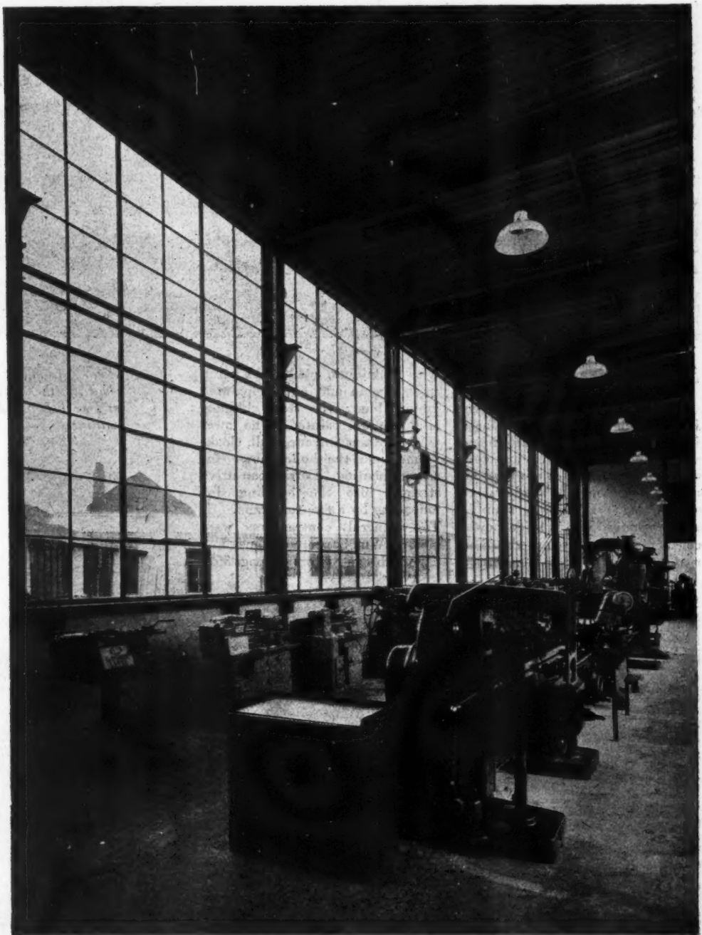
Above, interior of workshop showing the position of the bus-bars below window sill. Right, general view.
