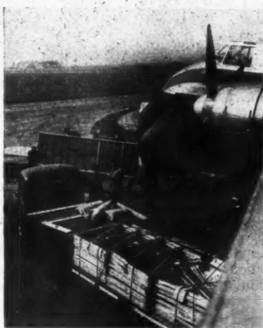
Sections of an aluminium pre-fab school, made by the Bristol Aeroplane Company (Housing) Ltd., being loaded for shipment from Weston-Super-Mare to Paris. The school has been erected in the Avenue Victor Hugo.
