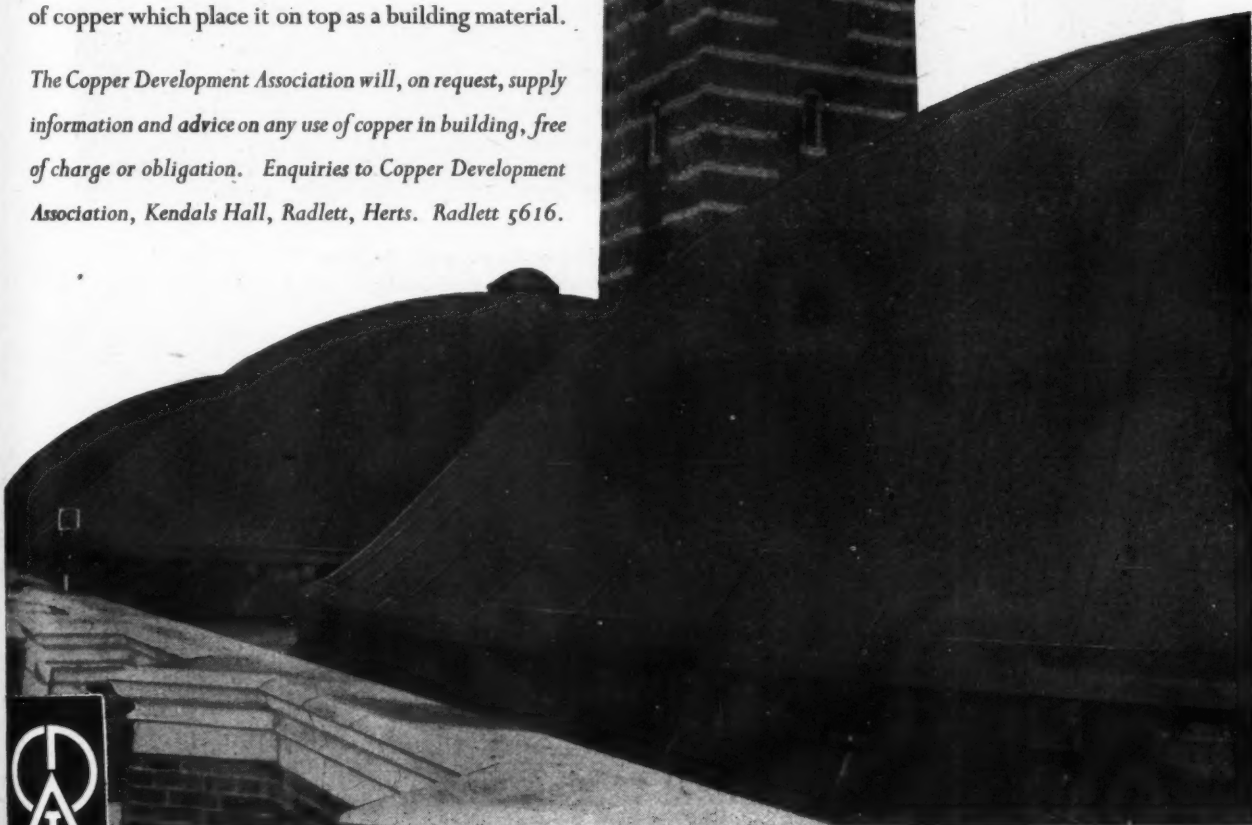
Westminster Cathedral domes roofed with copper
