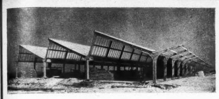
Left: the factory under construction, showing, on the right, the cantilevered rafters to the loading bay.
