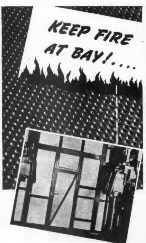
Illustration shows Section of Durasteel 3DF2 kolating Partitions and Doors between Trans-former Switch Units at Wolverhampton Genera-ting Station—Courtesy of West Midlands J.E.A.
