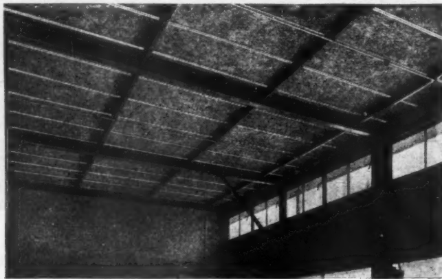
Temporary Shops, Ferensway, Kingston- upon-Hull, showing flat roofs of Thermo- coust Channel-rein- forced slabs. Andrew Rankine, O.B.E., A.R.I.B.A., City Architect.
