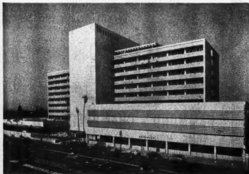
Precast stone facing on lightweight steel frame to building in Los Angeles. See 20.130.
