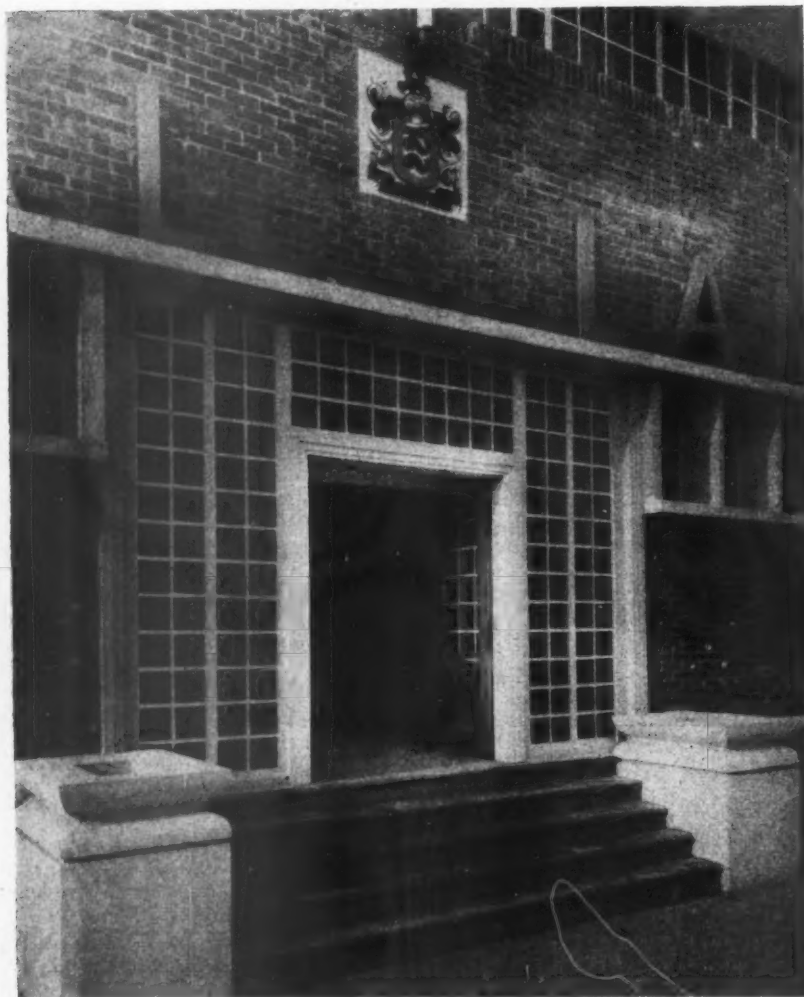
View of the main entrance showing the glass-brick surround to the main doorway.
