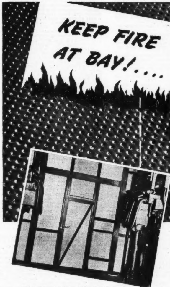
Illustration shows Section of Durasteel 3DF2 Isolating Partitions and Doors between Transformer Switch Units at Wolverhampton Generating Station—Courtesy of West Midlands J.E.A.
