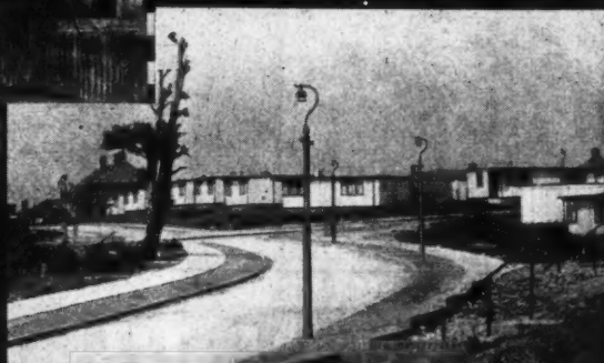
★ ADASTRA ★ HEXAGONAL LIGHTING COLUMNS 15 ft. MOUNTING HEIGHT
