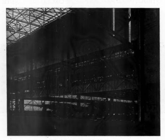
Flight shed doors, electrically lifted to give an opening of 30 ft. x 130 ft.
