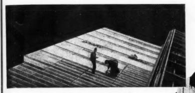
THERMACOUST Channel-reinforced Slabs are large, light weight, easily-handled units, with high heat-insulating properties. The reinforcement gives them exceptional structural strength. They are perfectly adapted for factory and office buildings. Leading Architects and Local Authorities are making extensive use of them for schools and municipal building. Limited quantities supplied without a steel authorisation. Standard slabs 6ft. long; 6ft. 8in. and 7ft. slabs made to order.
