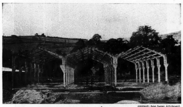
TRIPLE, SPAN FACTORY STRUCTURE CARRYING OVERHEAD TRAVELLING CRANE, RECENTLY ERECTED BY US AT MILFORD, DERBY
