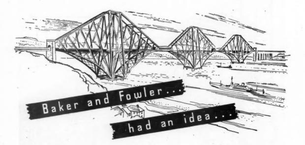
The outcome of their designing was the famous Forth Bridge with its cantilever construction and two large spans of 1,700 feet each. These brilliant engineers realised that the unusual features of the site demanded this novel treatment.
