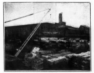
Aluminium Jib loading Prefabricated Aluminium House units for Export
