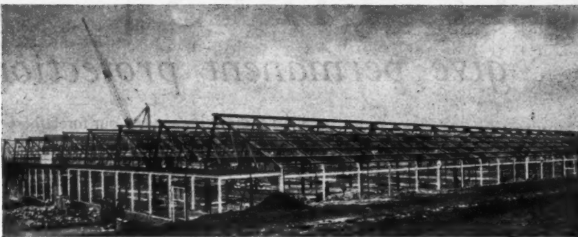
A factory with north light girder type roof and welded portal frames. Steelwork totals 850 tons.
