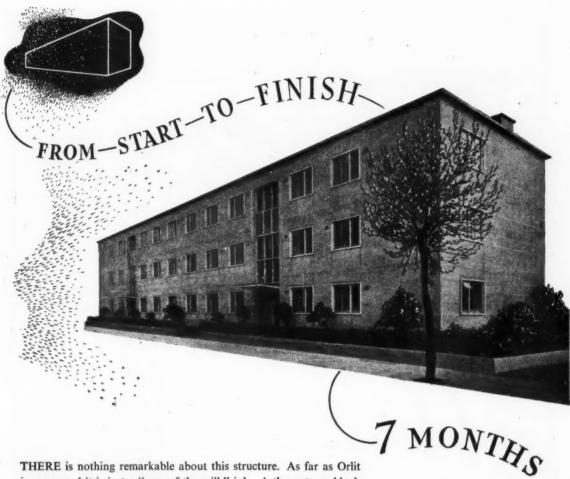
is concerned it is just a "run of the mill" job. A three-storey block of flats had to be built with the maximum speed and the minimum use of timber and steel. The Orlit pre-cast method of construction was the logical choice.
