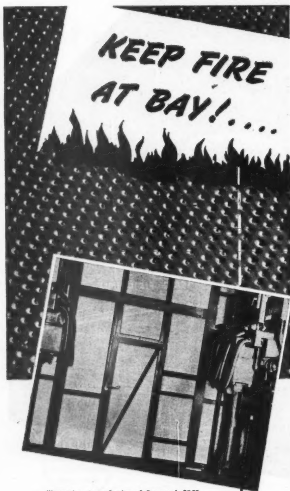
Illustration shows Section of Durasteel 3DF2 Isolating Partitions and Doors between Transformer Switch Units at Wolverhampton Generating Station—Courtesy of West Midlands J.E.A.
