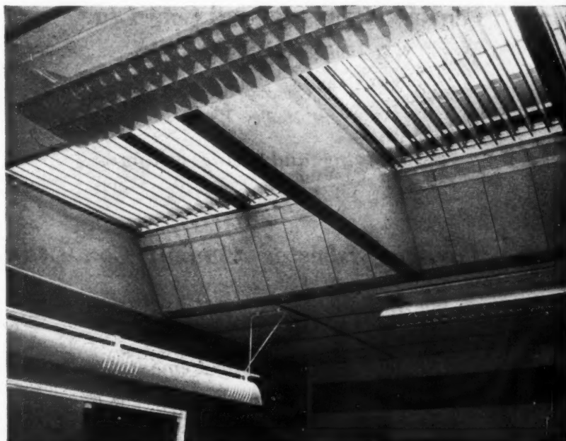
General internal view of ceiling, showing louvred frames and aluminium alloy shrouding to trusses.
