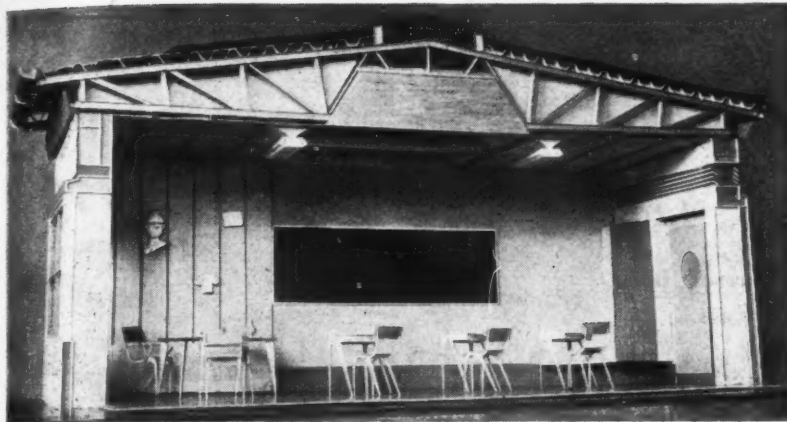
Sectional model of classroom showing detail of roof construction
