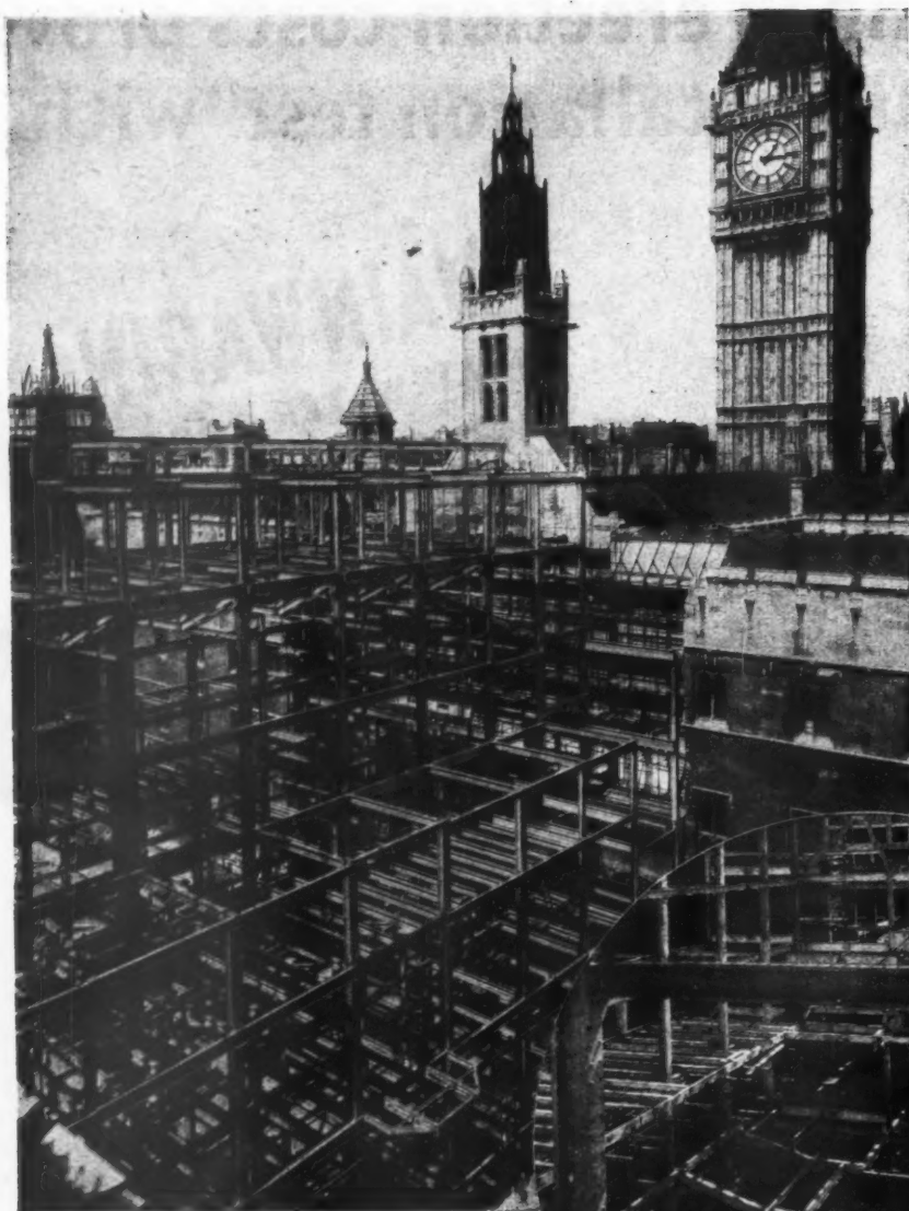
Structural steel in course of erection, for the House of Commons rebuilding. For the Ministry of Works.
