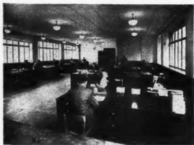
These Goods Offices at Canada Dock, Liverpool, have been designed by the Architects' Office of the Civil Engineer's Department, London Midland Region, British Railways. The building is steel framed, and is designed for future extension. A 3-ft. 4-in. grid has been used. A suspended ceiling to the beam soffits, together with walls which are flush with the stanchions, gives an unobstructed office space which allows for easy rearrangement of the plywood partitions.
