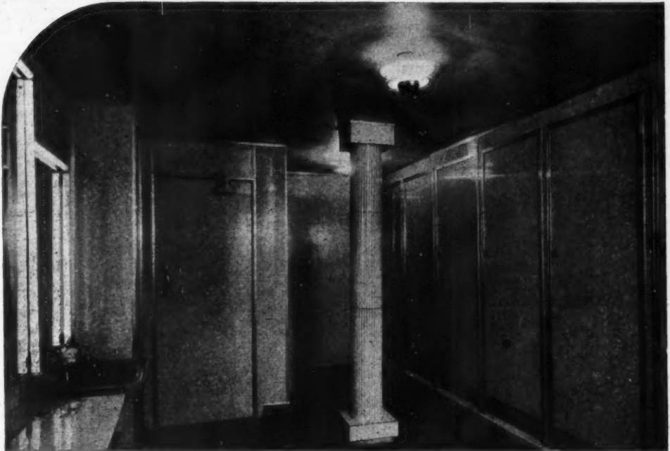
General view of Ladies' Toilet at London Palladium. Designed by Edwin Lawson, A.R.I.B.A. Fabrication with "Formica" faced "Holoplast" panels and aluminium.
