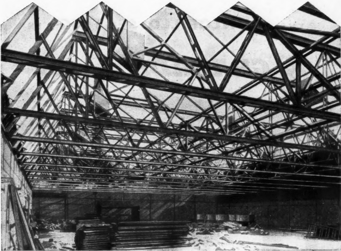
Warren girder roof, 85 ft. clear span
