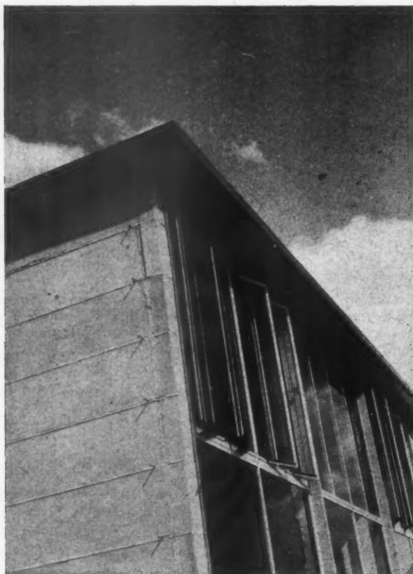
Detail of the eaves and wall finish at Essendon School (type I) for comparison with, above right, the eaves and wall treatment of a junior school (type II) at Little Green Lanes, Croyley Green. This latter school was part of the 1947 school building programme.
