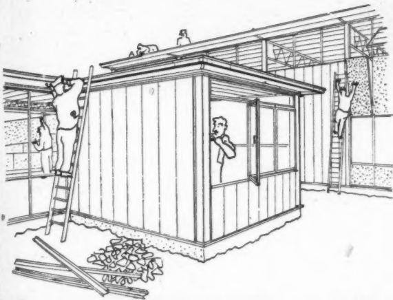
7. Metal fascias are fixed to the eaves and the bituminous felt roof covering dressed over them. Soffits are lined with asbestos. Window frames are screwed to the angle surrounds and the openings glazed or fitted with metal inserts consisting of two metal dished panels with glass silk filling.
