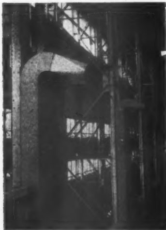
The aluminium ducts which discharge warm air into the assembly hall.
