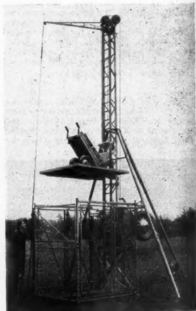
The Warry brick hoist with safety gates which is shown in model form at Olympia.
