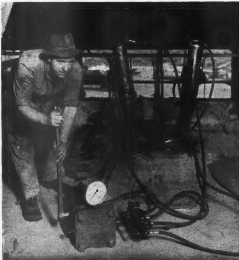
Post-stressing the reinforcement in the Lafarge Aluminous Cement stand. See page 576.
