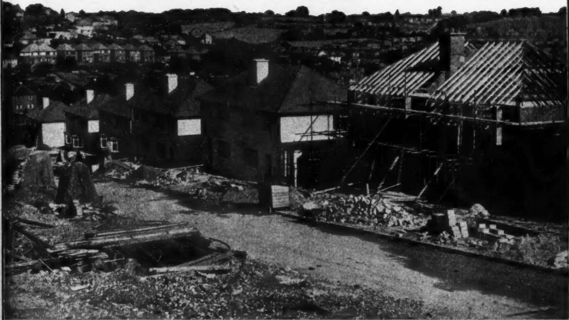
WIMPEY 'NO-FINES' HOUSES: THE DRAWINGS BELOW SHOW THREE MAIN STAGES IN THEIR CONSTRUCTION
