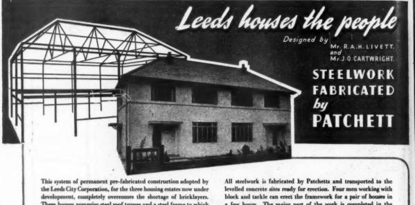
These houses comprise steel roof trusses and a steel frame to which vibrated pre-cast concrete units are fastened to form the outer wall skin.
