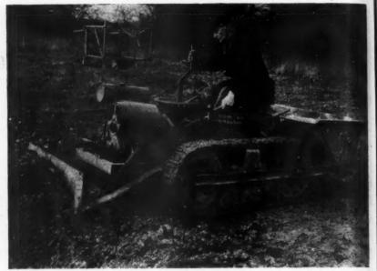
which is a standard agricultural machine slightly modified, can negotiate the roughest site and can dump the concrete right into its final position. The trial showed that the labour distributing the concrete could easily be halved but at the same time the output of the mixer could be doubled. For the small site it is always a problem
