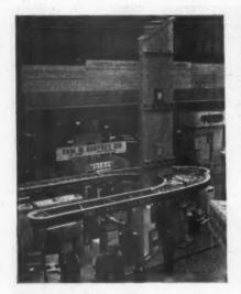
The Gas Council's stand, with its full-size replica of the gas-fire flue construction for a multi-storey building incorporating precast flue blocks.
