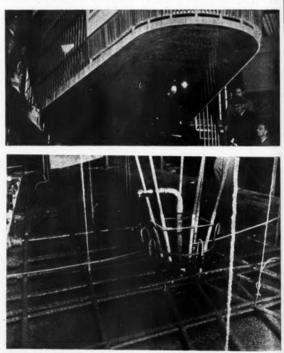
Details of the Lafarge Aluminous Cement stand. Top, the soffit of the finished slab showing the staining caused by the reinforcement. Below, the reinforcement during construction; the pipe, the head of which projects through the slab, is for water-cooling during the setting of the cement which reaches a high temperature.
