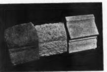
Left, an example of the work of the Universal Cleaning and Restoration Co. The model shows stages in the repair of decayed stone, which is cut back, keyed and holed for cramps, with the completed repair on the right. Below, two views of the Ascot Balanced Flue Multipoint Gas Water Heater, with and without cover. Bottom, the Kwik form shuttering for barrel vault roofing.
