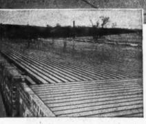
General view of Aluminium Decking prior to the application of Insulation Board and weather resisting surface.
