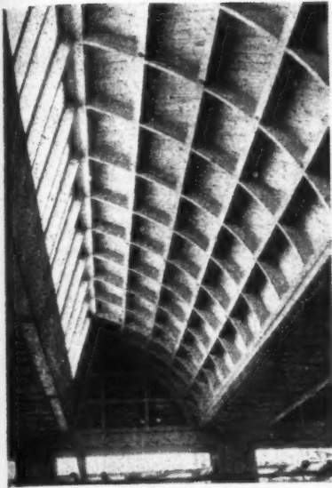
Swiss north-light roof of 65-ft. span in prefabricated glued timber construction. See 18.34.
