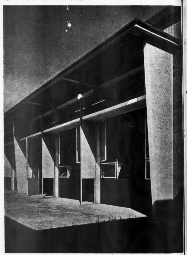
The south façade of a typical classroom showing canopies and baffles for light control.
