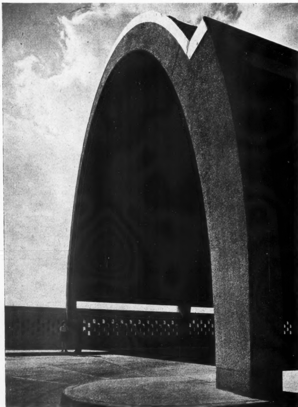
Detail of bus station arch, which is 30 ft. high and spans 60 ft.
