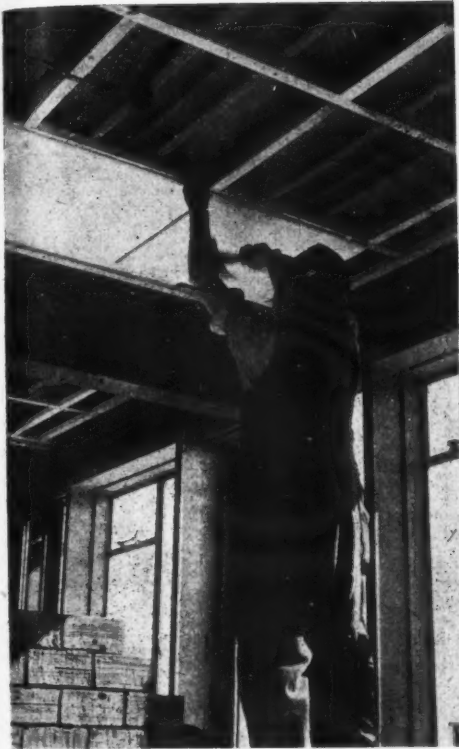
The internal lining of insulation board, sandwiched between asbestos sheets, being fixed in position.
