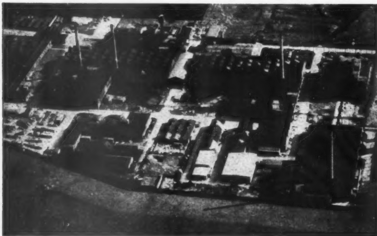
Factory for Messrs. International Alloys Ltd. Aylesbury. Consulting Engineers : Messrs. Malcolm Glover & Partners, Westminster, S.W.1
