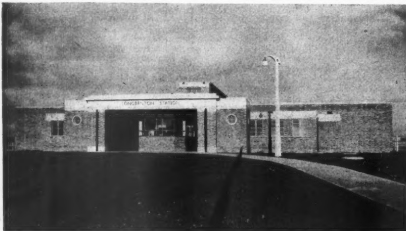
A new station has been built by British Railways at Longbenton, near Newcastle-on-Tyne. The buildings were designed by A. N. Thorpe, architect in the Civil Engineer's Department of the NE Region. The station accommodation consists of circulating area, and two platforms, with a ticket office controlling the entrance barrier. Waiting rooms and lavatories are also provided. The buildings are planned to permit future extensions to deal with increased traffic when the surrounding residential area is completely developed.
