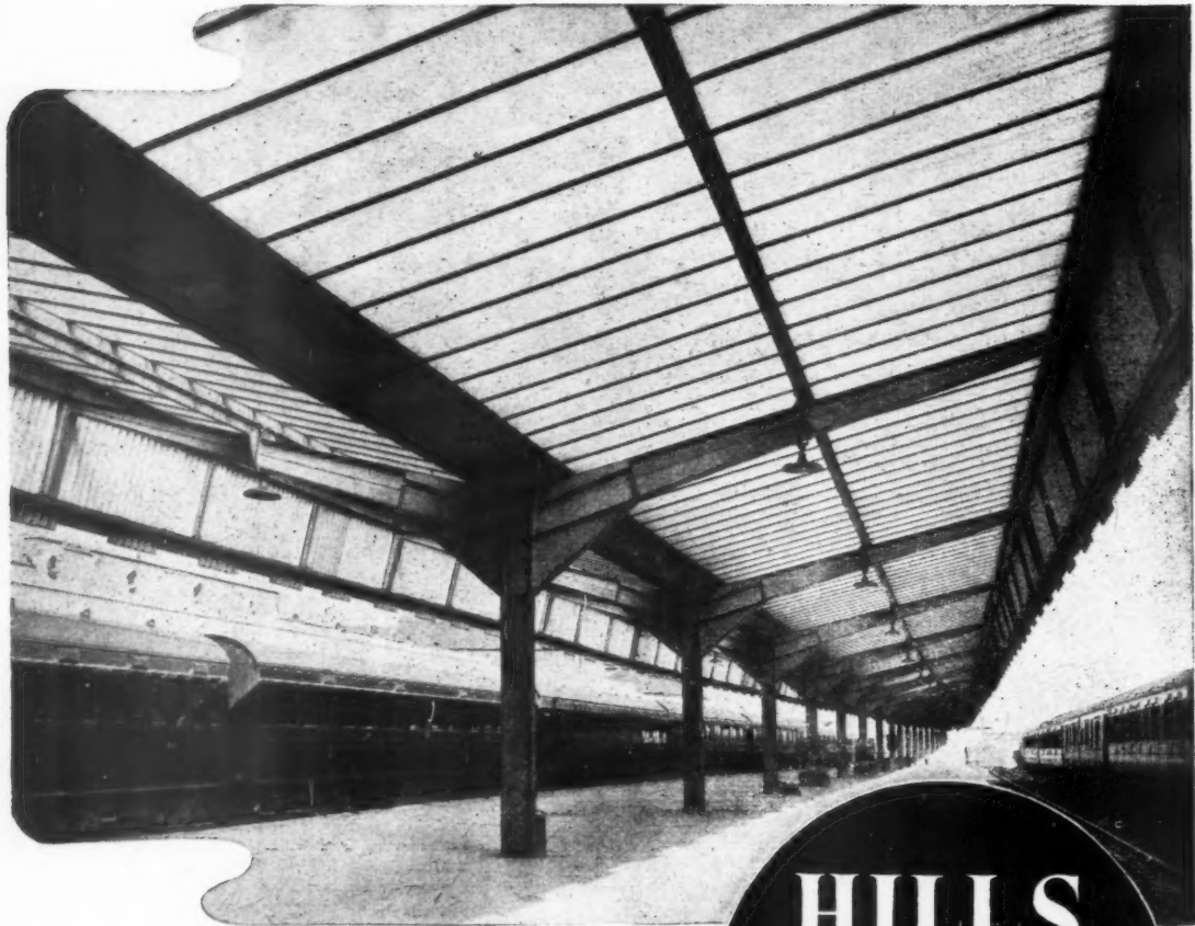
Hills Patent Glazing at York Road Station, Belfast, for the Northern Counties Committee. Engineer: N. C. Cain, B.Sc.
