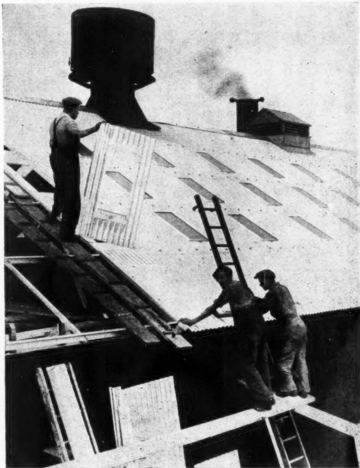
Re-roofing a factory with aluminium trusses and patent sheet roof-lighting.
