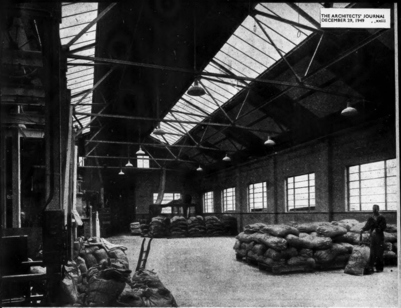
Loading Bay at the works of MESSRS. LATHAM & CO. Bromborough.
