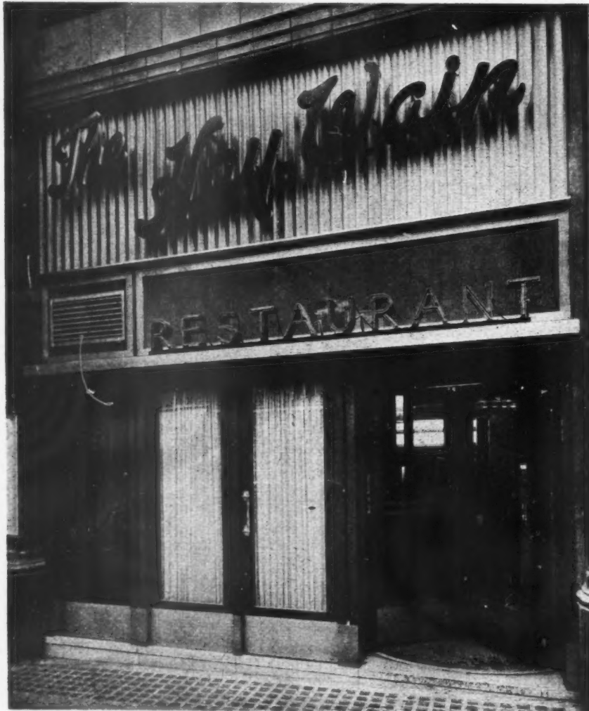
Left, the main entrance from the Haymarket. Bottom: left, the entrance lounge seen from the bar; right, the entrance lounge.
